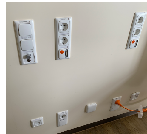
Referenz Elektroanschlüsse Kopfende Patientenzimmer Station A2
