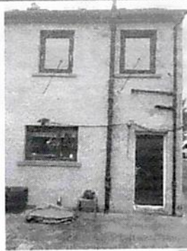
REAR OF PROPERTY Scaffolding required
