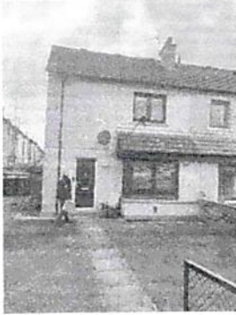
FRONT OF PROPERTY Scaffolding required
