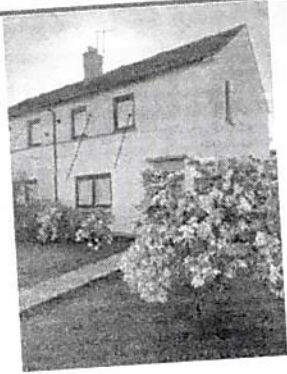
FRONT OF PROPERTY Scaffolding req
