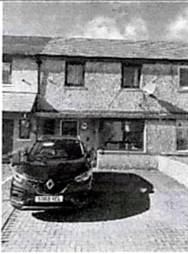
FRONT OF PROPERTY Scaffolding required
