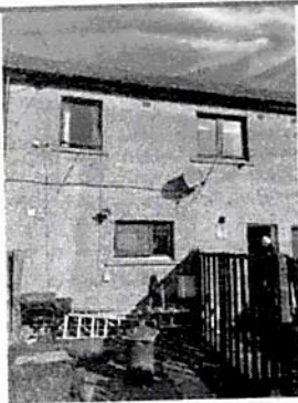
REAR OF PROPERTY Scaffolding required
