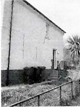
SIDE OF PROPERTY Scaffolding required
